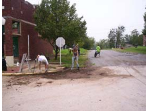
Workers unearth long forgotten curb.
