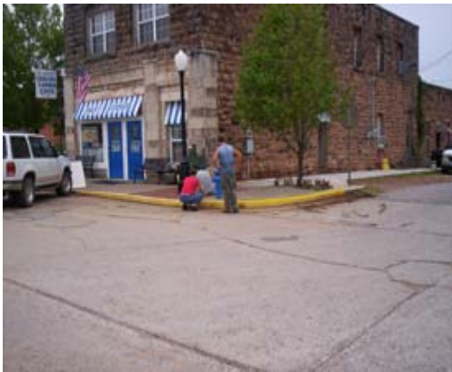
Karin Goins and sons Ron & John paint curbs.
